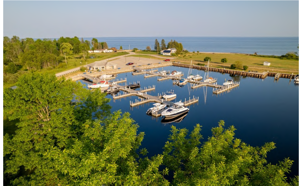
Aerial view of the docks and recreational watercrafts at the marina at J.W. Wells State Park in Cedar River, MI. Photo: Tyler Leipprandt and Michigan Sky Media LLC in cooperation with the MI DNR.
